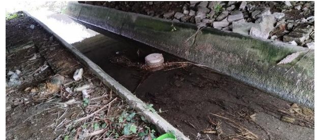
7 A1303 Bridge Channel
